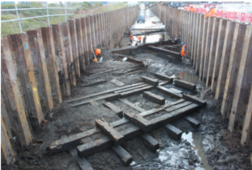
Fig. 2: Thames Ironworks uncovered at Instone Wharf.
